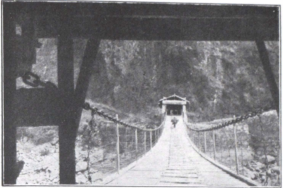
Mules crossing the Mekong suspension bridge.
